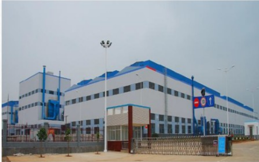
New Foundry Phase 1
