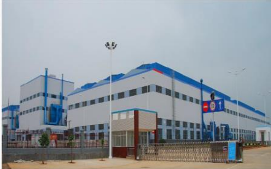
New Foundry Phase 1
