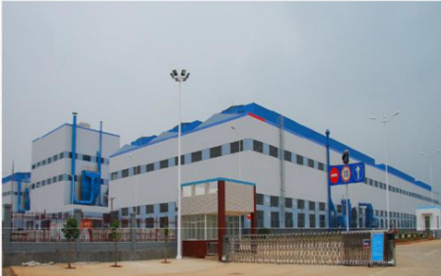
New Foundry Phase 1
